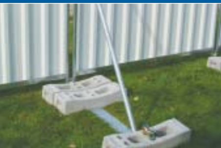
Strut design including concrete bases
